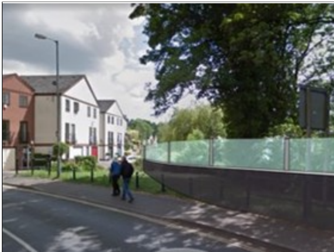
Figure 3: Part of the proposed flood alleviation scheme at Beales Corner, Bewdley. See Annex A, Table A2, item P1 for more information on the development of the scheme.
