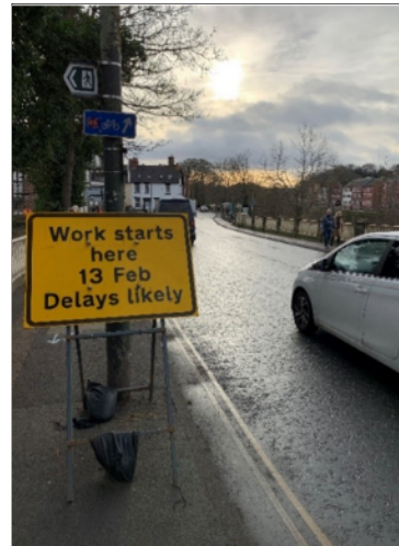
Figure 4: Tree works were done in early 2023 to enable the scheme construction to follow on later in the year
