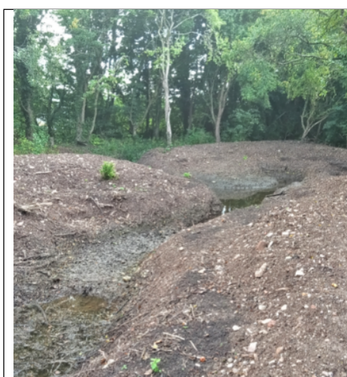
Figure 14: A newly constructed storage pond at Padgets Lane, Redditch. To add ecological value it was designed to permanently hold water at low levels. (Annex A, Table A1, item C7 refers.)
